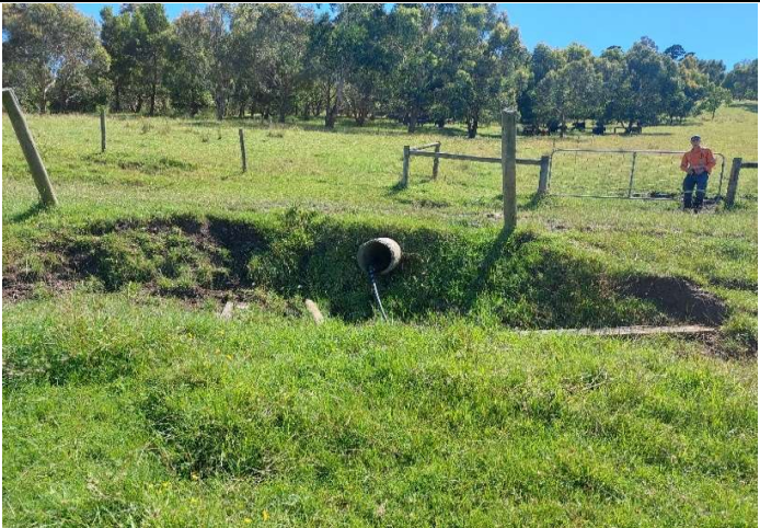
Plate M17-D Pipe culvert under access track
