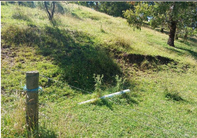
Plate M02-C PVC overflow line from Spring 02 and slump above
