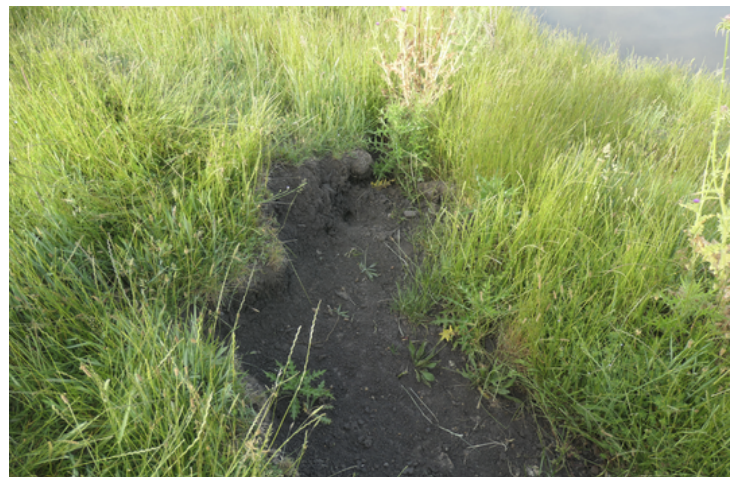
Dam 13 - looking east (erosion)
