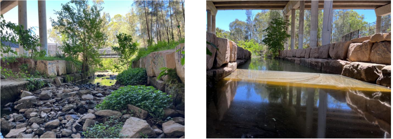
Figure 9: Upstream (left) and downstream (right) photos from AE6
