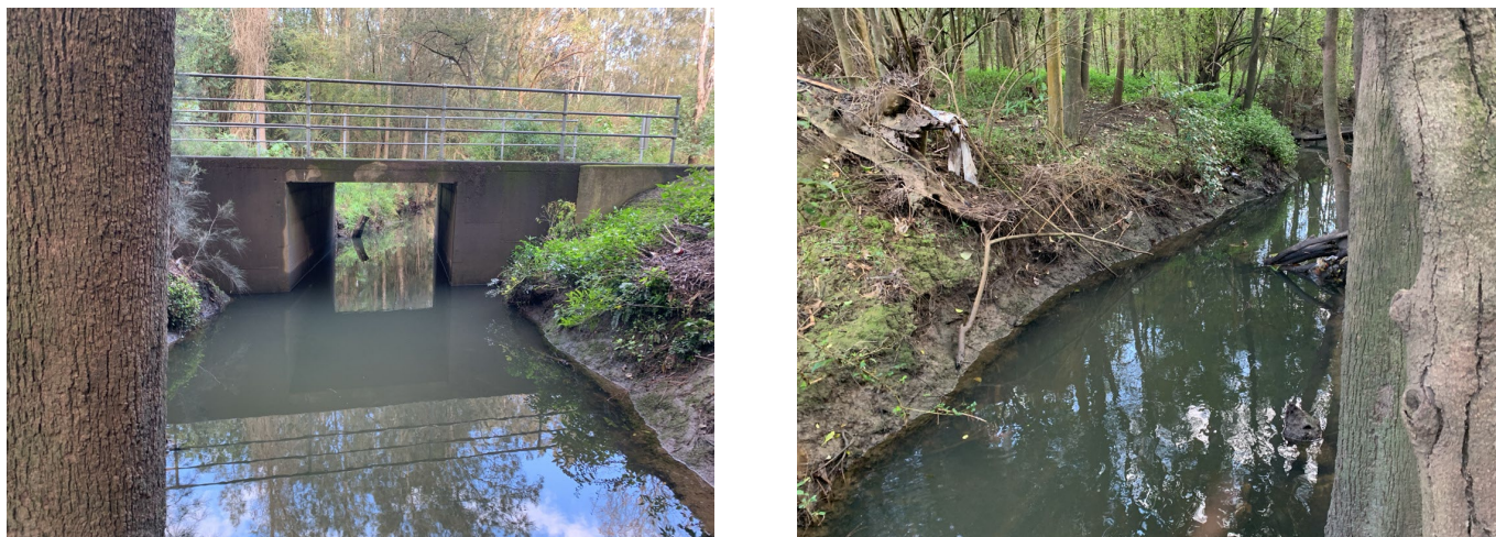
Figure 5: Upstream (left) and downstream (right) photos from AE3
