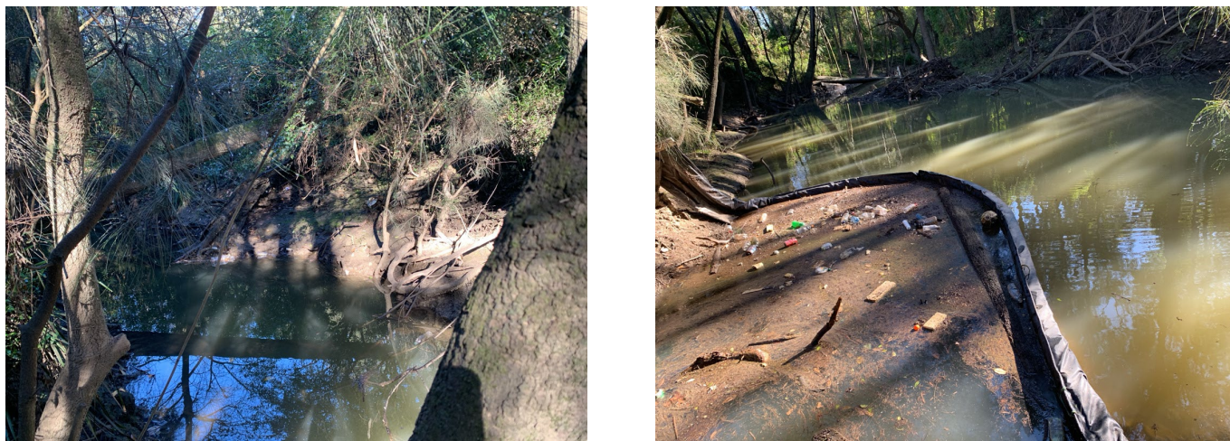
Figure 6: Upstream (left) and downstream (right) photos from AE4
