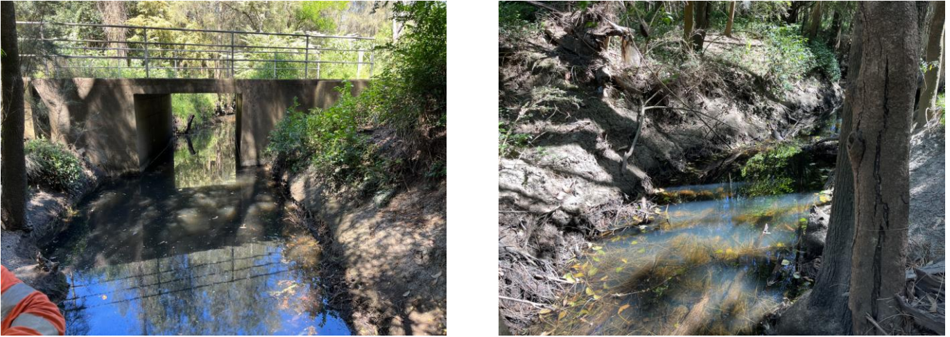
Figure 6: Upstream (left) and downstream (right) photos from AE3
