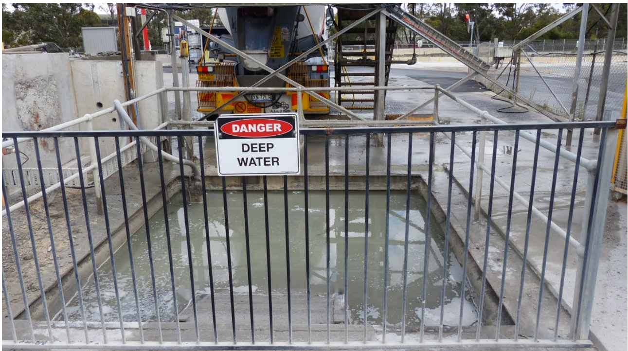
Photograph B.8 Concrete washout area
