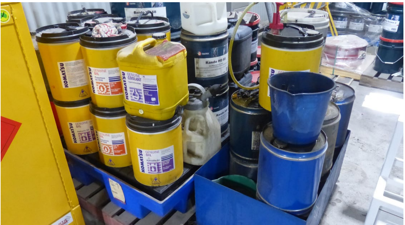
Photograph B.6 Bunded chemical storage area
