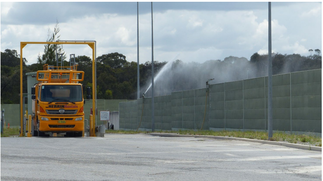
Photograph B.11 Dust suppression sprinklers
