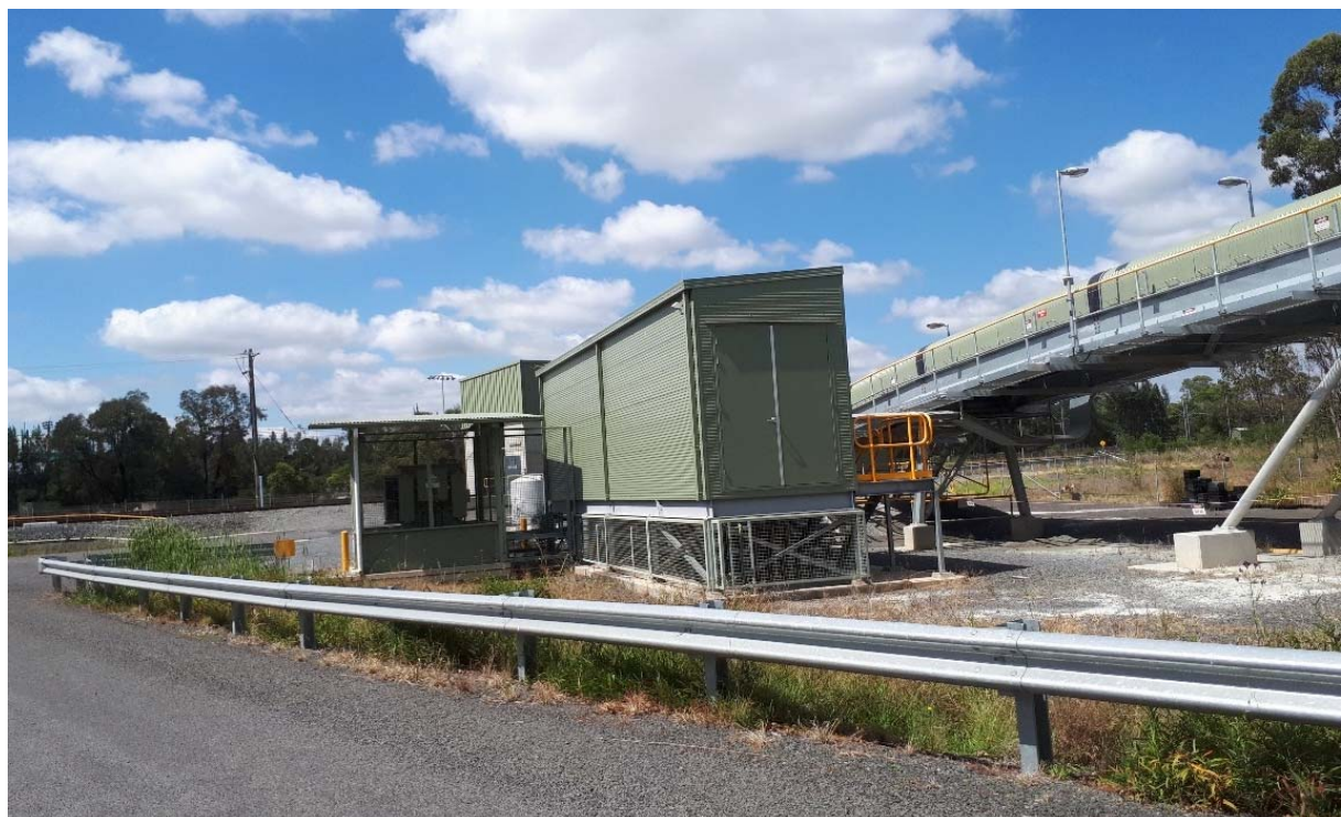
Photograph 3.11 Covered conveyor belt that transports aggregates from the rail facility to the RHDC
