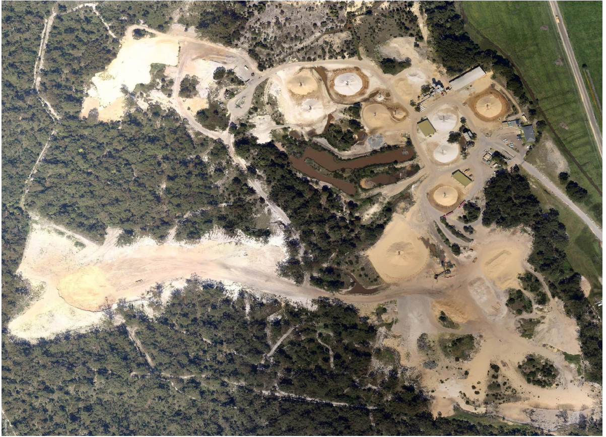
Overall view of Salt Ash Site
