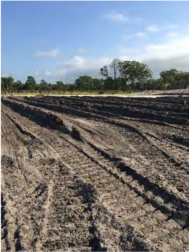
Figure 3 Top Soil Replacement
