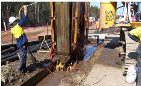
finished in poor conditions such as heavy downpours. This required mix adjustment on the spot in order to maintain water-to-cement ratio specification with wet sands and water entering the agitator in transit.
