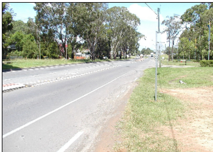
Figure 1 Knox Rd / Nurragingy Reserve access intersection – looking south
