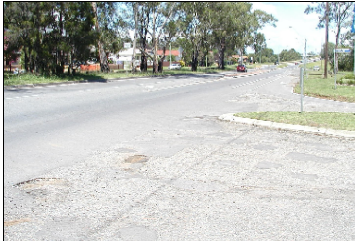
Figure 2 Knox Rd / Nurragingy Reserve access intersection – looking south from Reserve access approach
