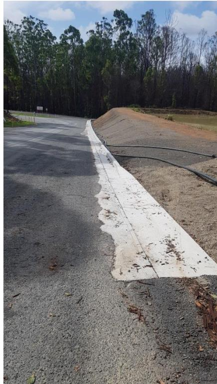
**Photo 3 Kerbside drain and gutter installed at the main Jandra Quarry driveway**
