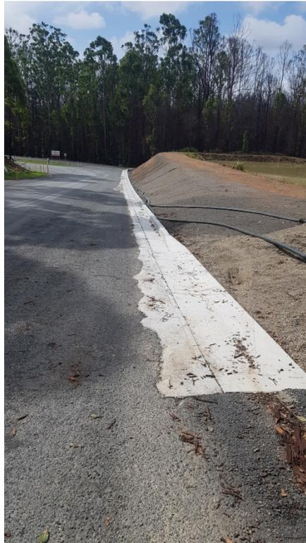
**Photo 2: Kerbside drain and gutter installed at the main Jandra Quarry driveway**
