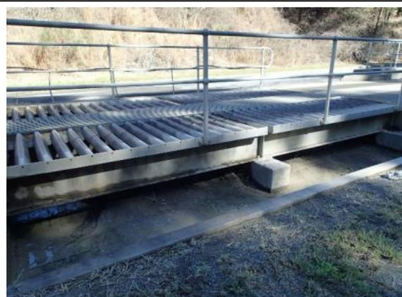
Shaker system at the site exit, which trucks pass over following the wheel wash. Excess water is drained and cycled through the wheel wash, while material is collected for disposal
