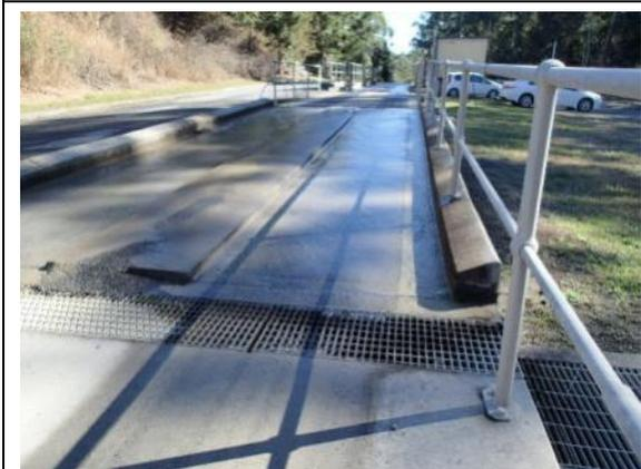
Wheel wash system at the site exit, with water cycled through via a pump before draining to the Main Dam for reuse.
