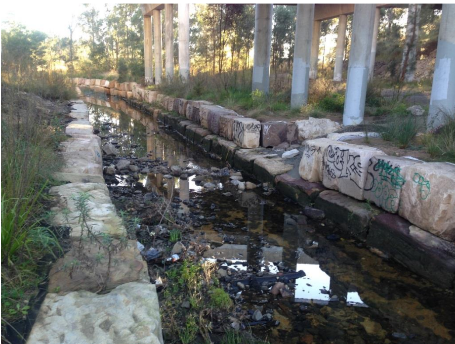
Photo 6 : Site AE6 showing fully stabilised creek banks with sandstone rock armouring
