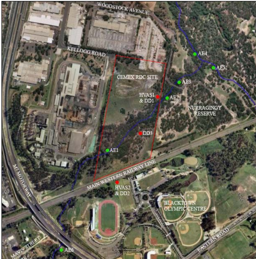
Figure 1 - Air, water and aquatic ecology sample locations map (Source: Google Earth satellite imagery)
