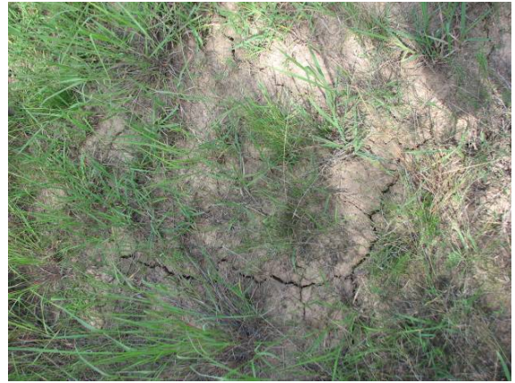
Photo 18 - Cracking soil near SH4
