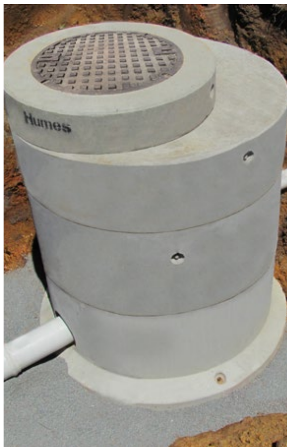
Left: Access chamber structure ready for backfilling
