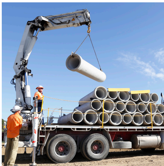
Top: Concrete pipe delivery
