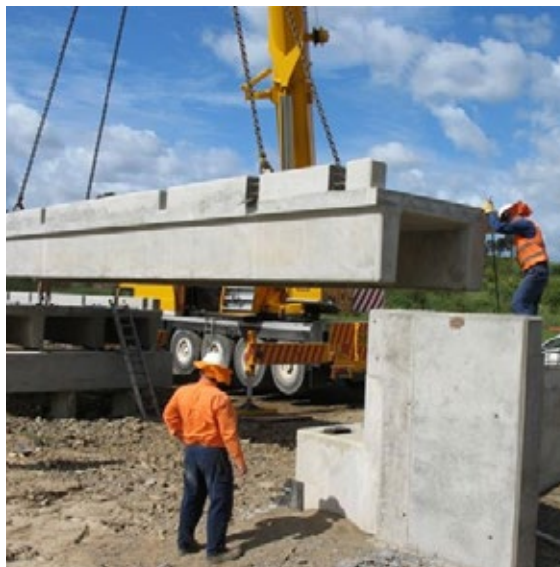
Top: Placing a deck and girder unit onto an abutment
