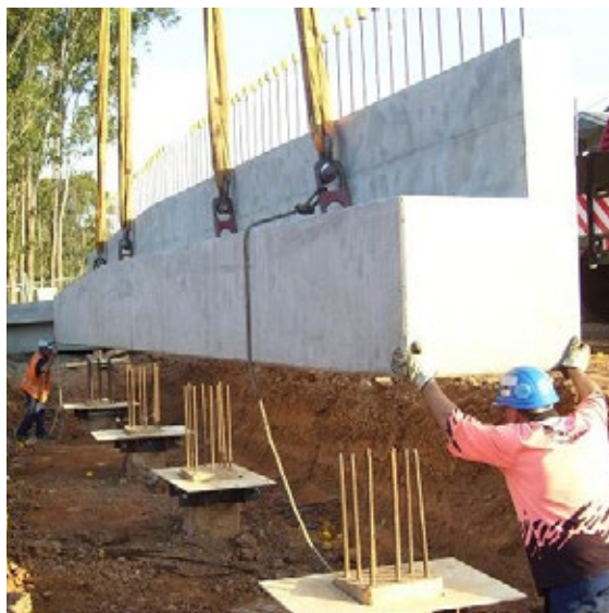
Top and bottom: Placement of headstock/ abutments onto piles
