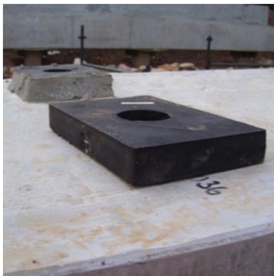
Top: Placement of elastomeric pads
