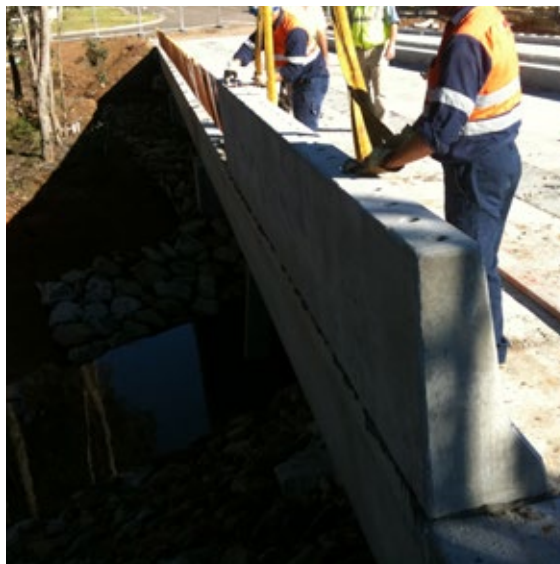
Top and bottom: Fixing concrete barrier onto deck
