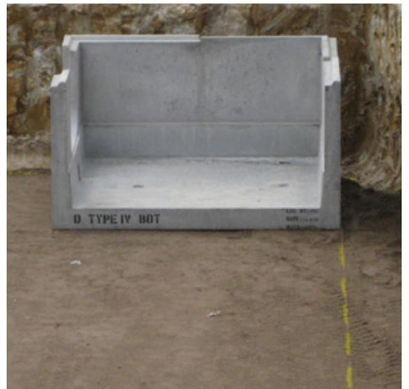
4. It is essential to ensure all bottom pieces are level (check using a spirit level across the diagonals) and square with the perimeter markings before the anchors are removed. This will minimise any gaps when the top pieces are installed, forming the module.
