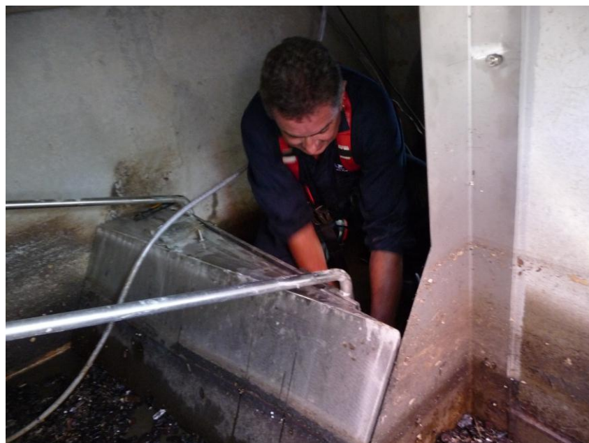
Figure 4 – Installing the hoses for the Automatic Samplers
