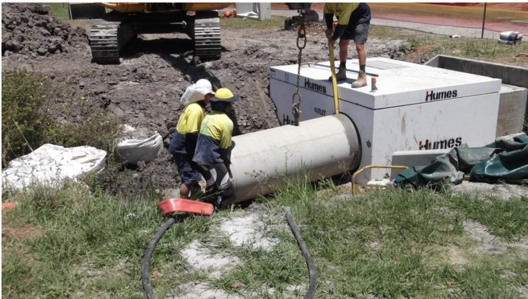
Figure 1 – Humegard® HG27 Installation at USC
