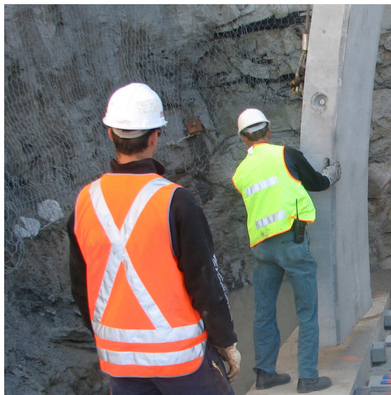
Left: Humes site representative observing installation
