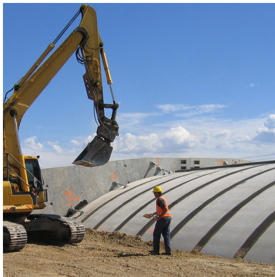
Top: Joints sealed, checking backfill
