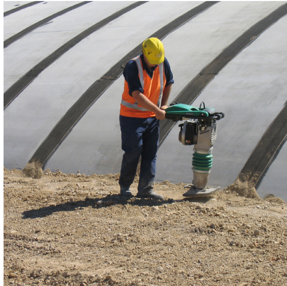
Left: Hand compaction of backfill
