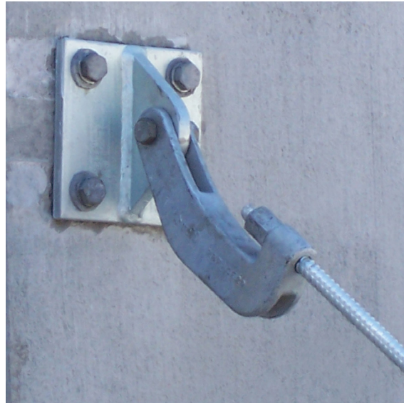
Top: Spandrel connection
