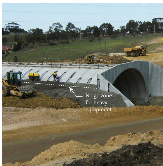
Left: Observe the no go zone for heavy equipment
