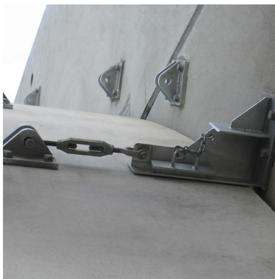
Left: Temporary installation bracket fixed into special end arch unit
