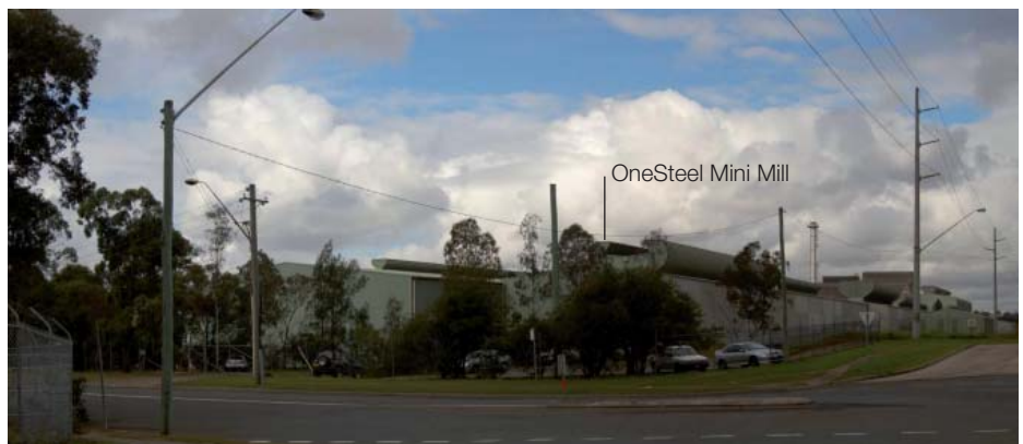
Figure 4.3.1 - View of One Steel Mini Mill site, looking south from Kellogg Road
