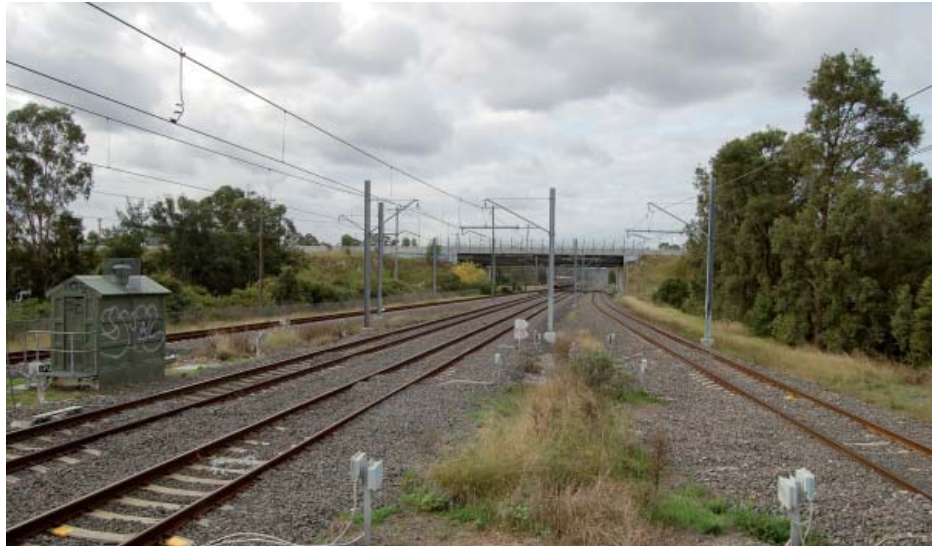
Figure 4.3.5 - View of Rail Corridor, looking east towards M7 Motorway
